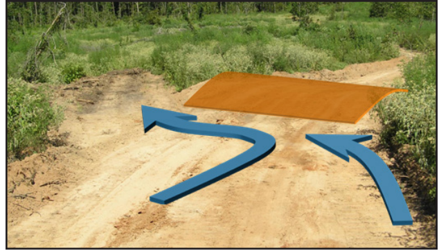
Figure 50. Waterbars and wing ditches help to safely drain road surface runoff water to prevent erosion. (Photo courtesy of the Texas Forest Service.)
