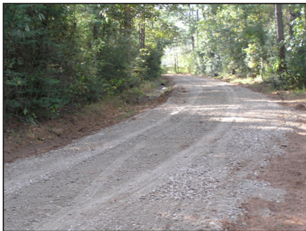
Figure 49. Armoring road surfaces can prevent erosion and improve accessibility. (Photo courtesy of the Texas Forest Service.)
