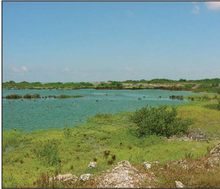
Figure 40. Constructed wetland in Texas. (Photo courtesy of the South Texas Environmental Institute, Texas A&M University-Kingsville.)
