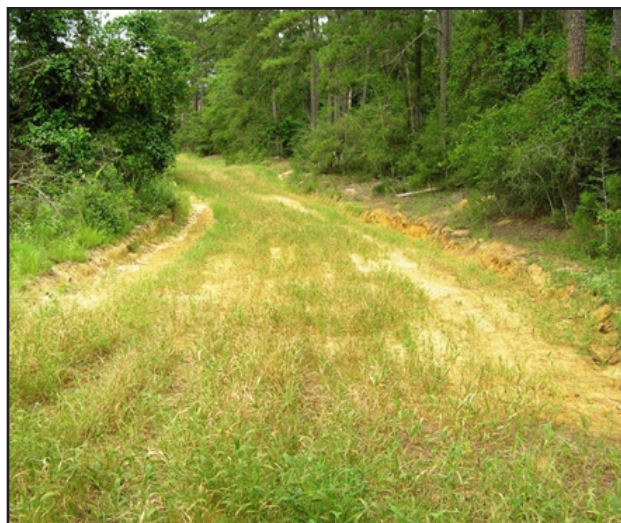
Figure 47. Revegetation stabilizes disturbed soil and prevents erosion. (Photo courtesy of the Texas Forest Service.)
