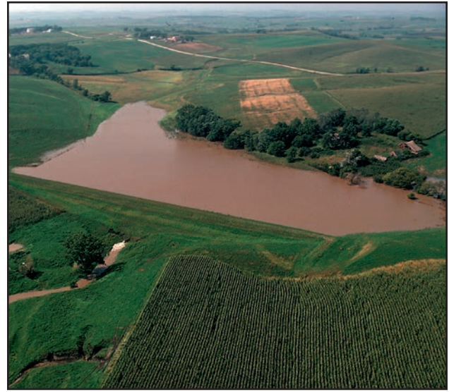
Figure 34. Water and sediment control basins hold runoff water to prevent flooding and sedimentation. (Photo courtesy of USDA Natural Resources Conservation Service.)
